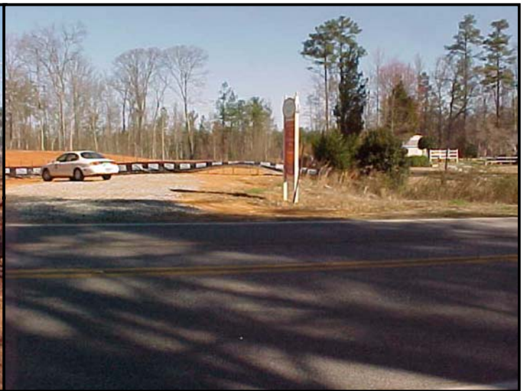
Looking at entrance from interior
