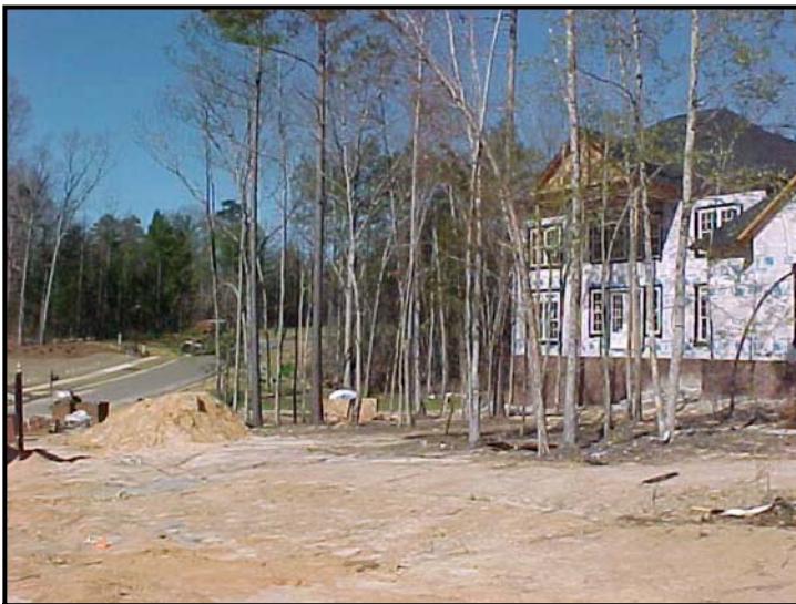
Looking at site from Laurent Way
